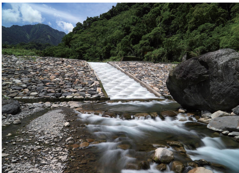
▲Figure 2-29 Improvement work at a check dam upstream of the Changjung Bridge at Wushikeng River in Taichung
