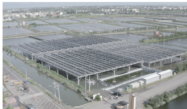
▲Figure 2-14 Solar panel fish farm
