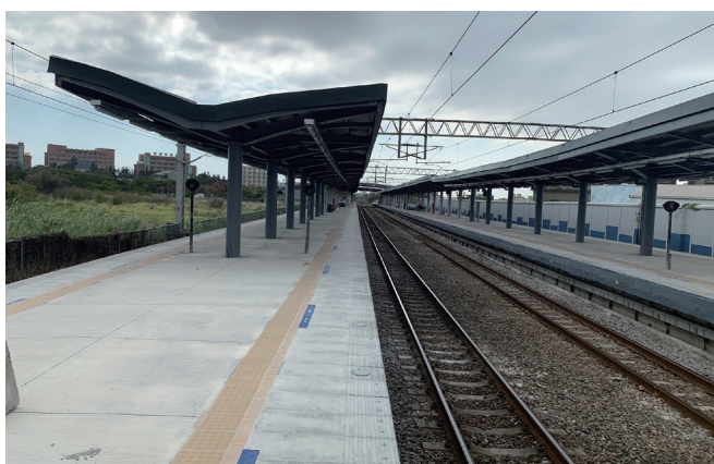
▲Figure 2-18 Platform alignment work at Peihu Station
