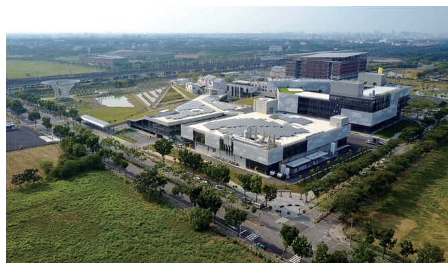
▲Figure 2-13 Shalun Green Energy Technology Demonstration Site
