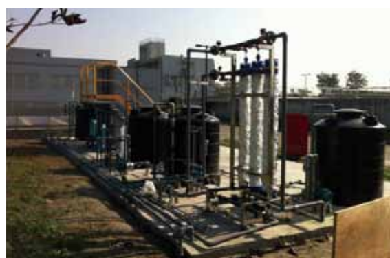
Ⓔ Erlin Sewage Treatment Plant: effluent water provides Erlin High School with Secondary domestic water.
