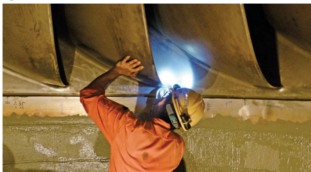
▲ Feitsui Power plant repairing (internal turbine inspection)
