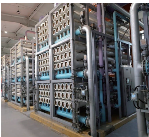
▲ Image 15 / Fengshan River Reclaimed Water Treatment Plant RO (Reverse Osmosis) Processing Unit
