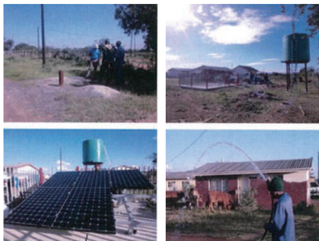
▲ Image 18 / Assisting set up of solar photovoltaic pumping systems in eight middle schools
