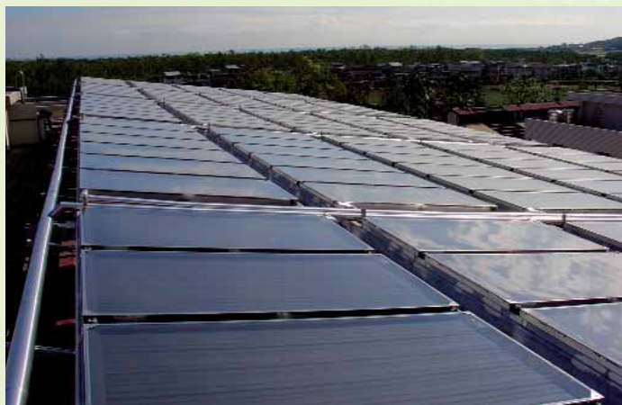
■ Solar thermal collectors installed on a roof at Dahan Institute of Technology (total area of 356m 2 )
