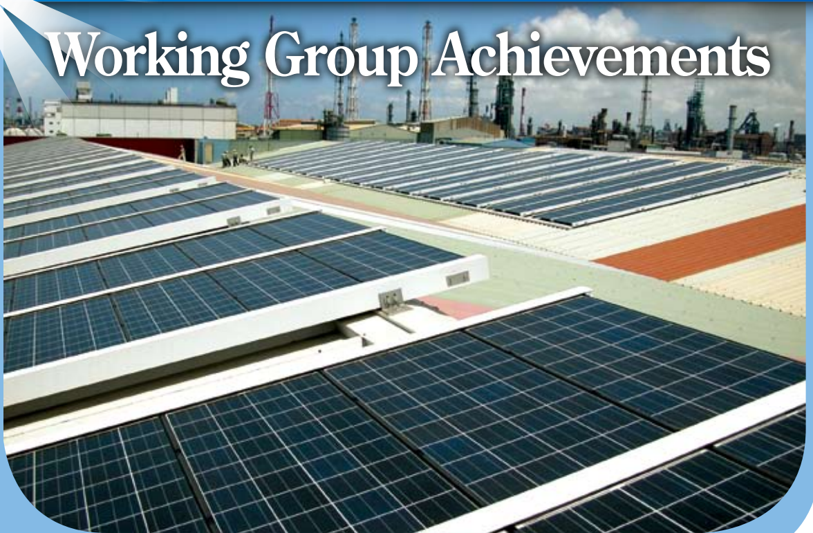
↑ 208kWp PV System of I-Domian Industrial Co., Ltd. in Kaohsiung
