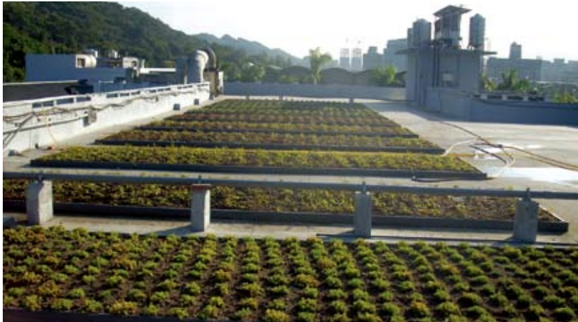
Shih Chien University green roof project to provide better insulation from outdoor heat
